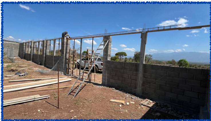
CONSTRUCTION OF THE WALL AROUND OUR PROPERTY
